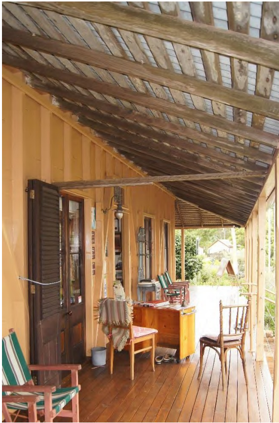
Figure 25: North eastern side of verandah (front entrance) showing unlined opened verandah with original shingle battens and rafters (AHS, 2019).
