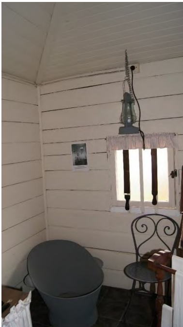
Figure 56: Bathroom looking at the western most corner showing wall boards, vinyl flooring and casement window (AHS, 2019).
