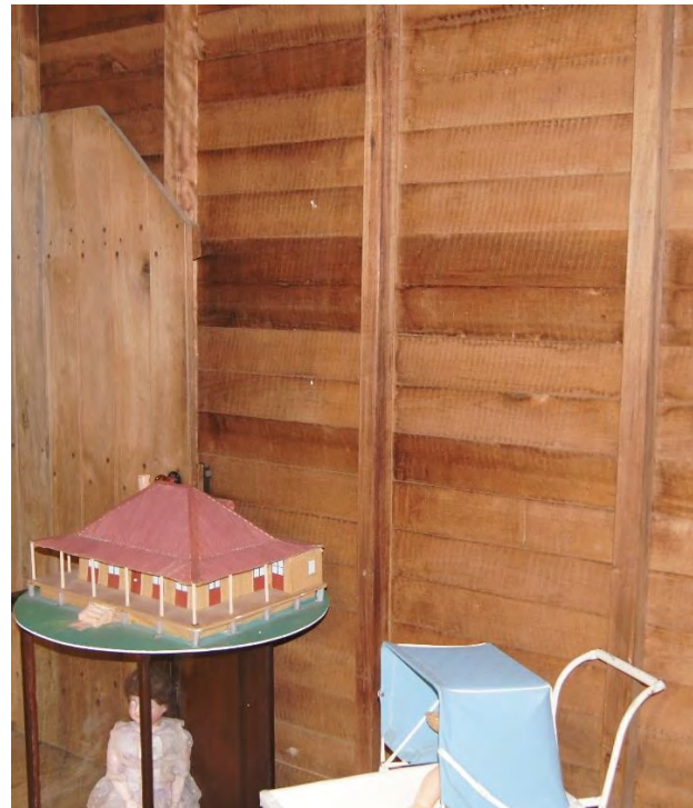
Figure 66: Exposed studs on the stairway's north western wall (AHS, 2019).
