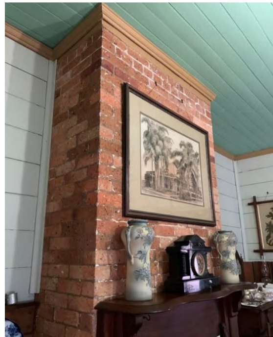
Figure 46: Original brick chimney/overmantel of the fireplace (AHS, 2019).
