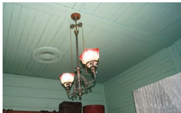
Figure 49: Ceiling showing partition wall division, ceiling rose and converted gas lighting (AHS, 2019).
