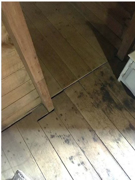
Figure 65: Wall stud of attic joined to lower floor wall stud (AHS, 2019).
