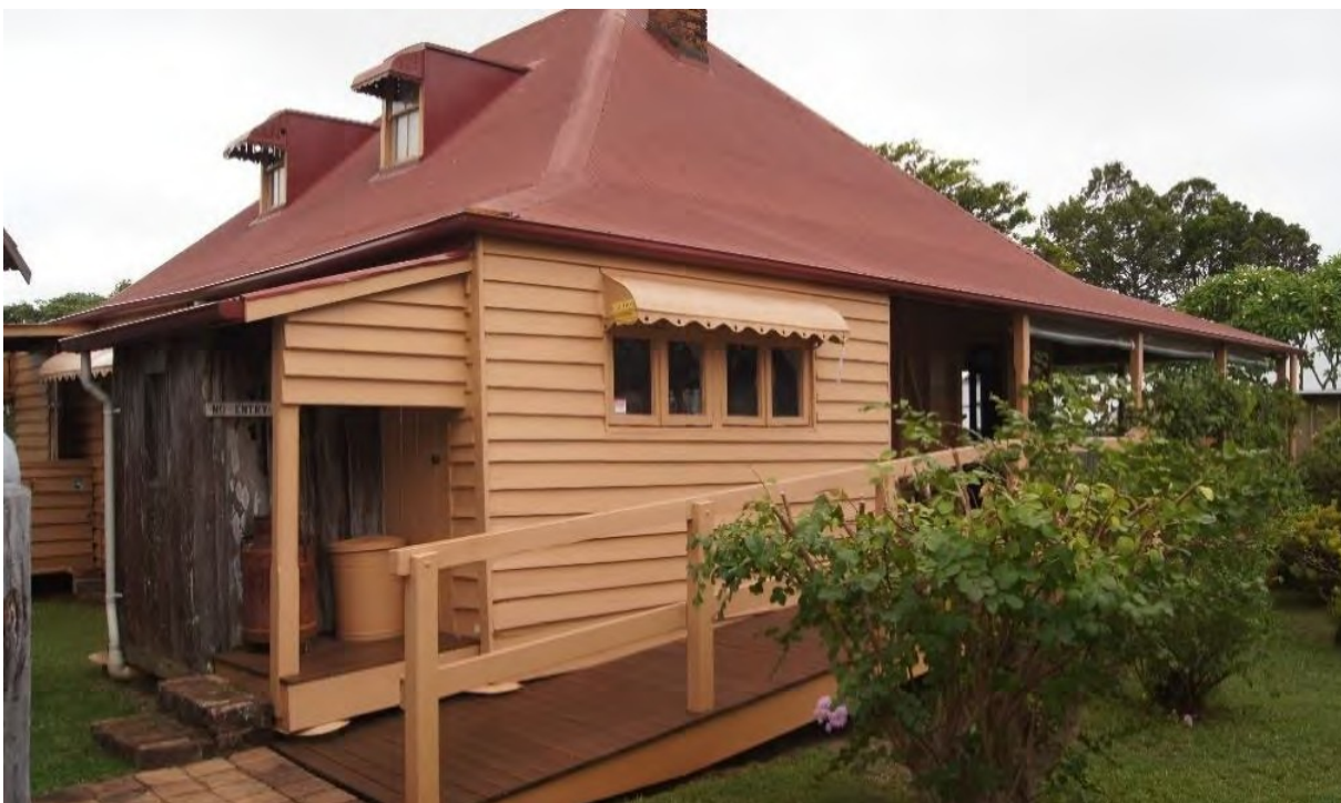
Figure 33: Eastern corner of the enclosed verandah showing weatherboarded kitchen area, early casement windows with 1930s hoods, and kitchen room extension with landing (AHS, 2019).
