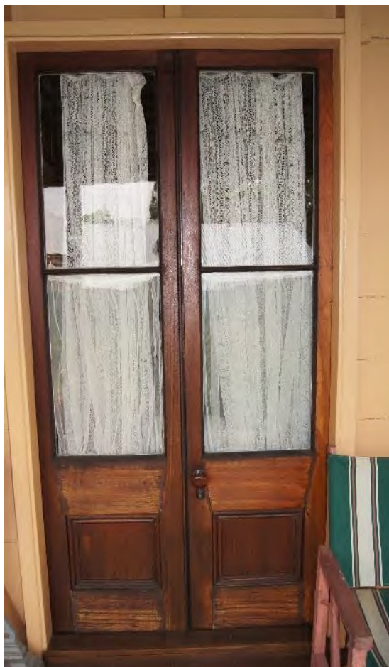
Figure 28: Original low-waisted timber and glass panel French doors (AHS, 2019).
