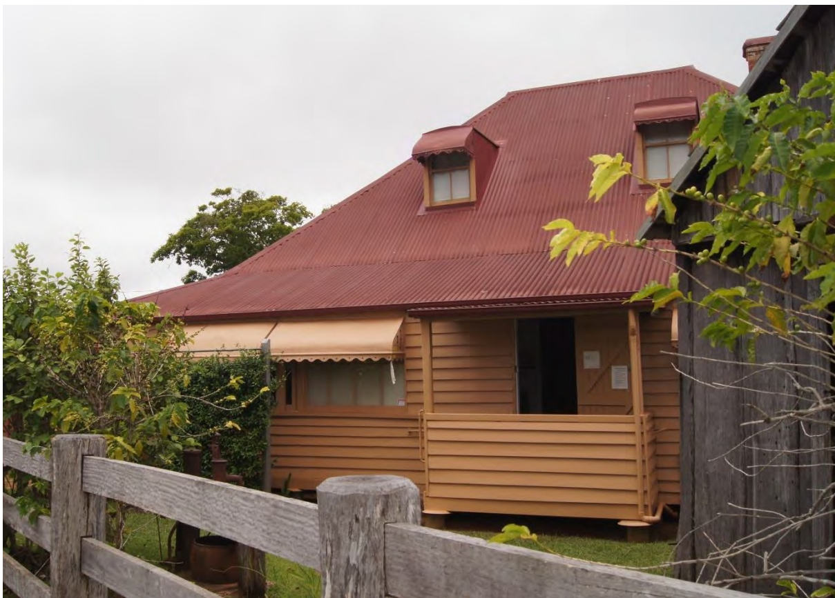
Figure 32: South western side of the cottage showing enclosed weatherboarded verandah, sash windows with hoods, and back landing (AHS, 2019).
