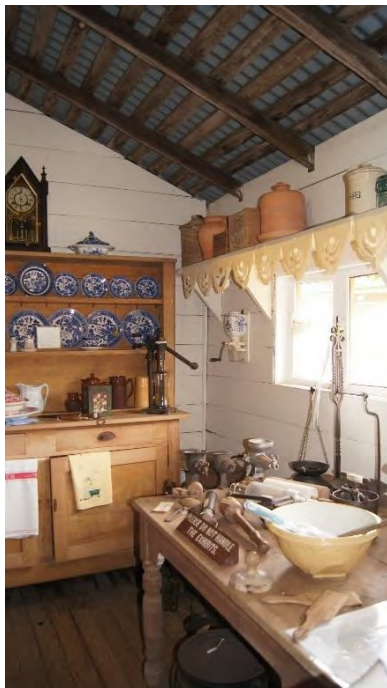
Figure 52: Kitchen looking at the eastern corner showing floorboards, wall boards and unlined ceiling with shingle battens and rafters (AHS, 2019).
