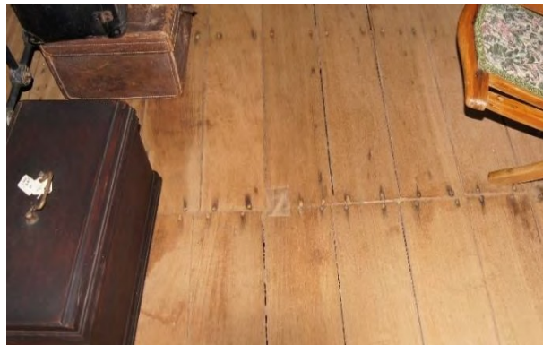
Figure 48: Original floorboards showing joinery for partition wall division and wall studs (AHS, 2019).
