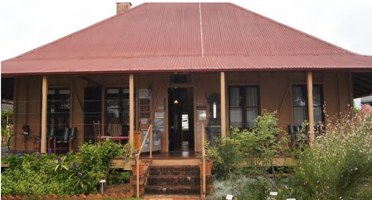
Figure 27: North eastern elevation showing front entrance of the core building with horizontal tongue and groove boards and external cross bracing, (AHS, 2019).
