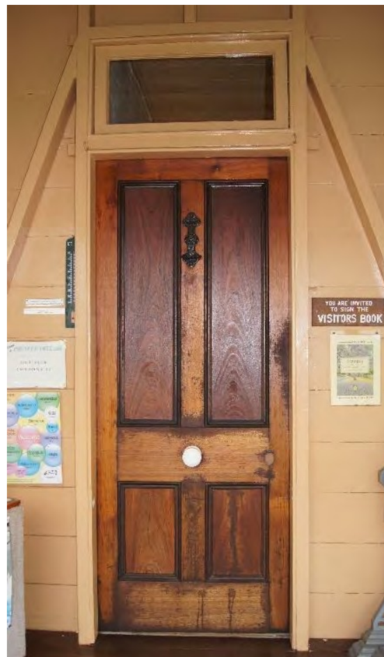
Figure 29: Original low-waisted, four-panel timber front door with glass transom window (AHS, 2019).
