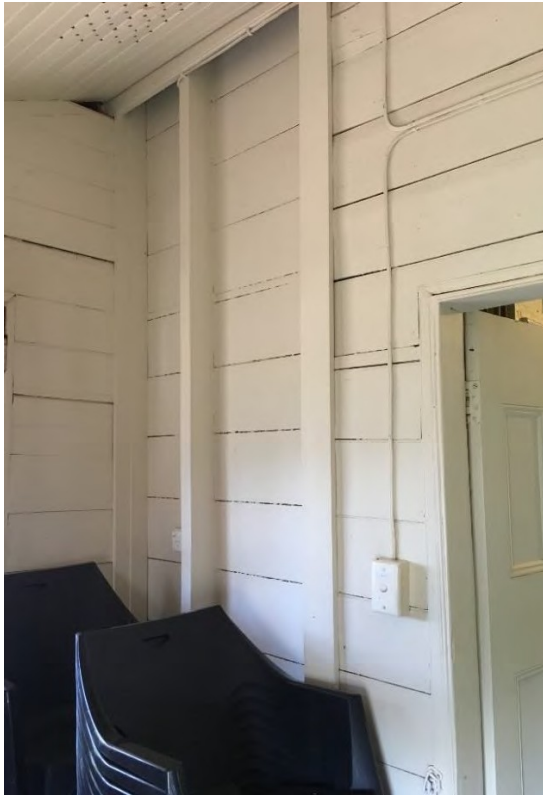
Figure 55: Bathroom showing the original external bracing and single skin construction of the core building along the south eastern wall (AHS, 2019).
