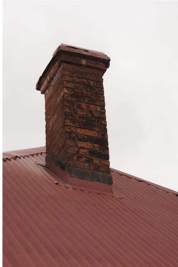
Figure 26: Original brick chimney with contemporary iron chimney cap (AHS, 2019).
