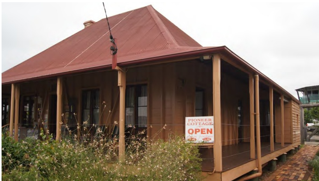
Figure 24: Northern side of the verandah showing stop chamfer timber posts, decking, pitched verandah roof, and wire balustrading (AHS, 2019).
