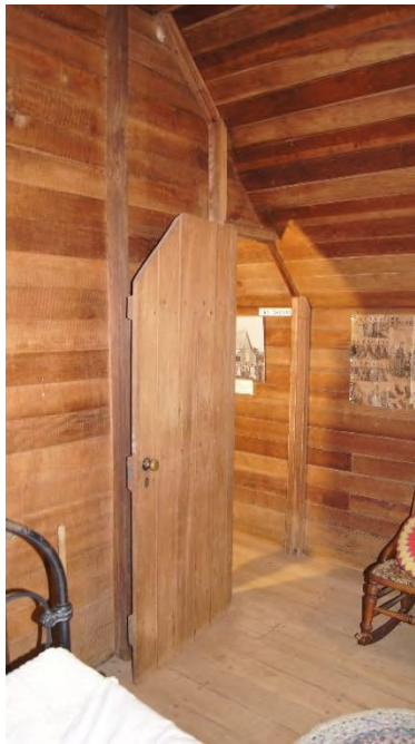
Figure 62: Timber boarded door separating the stairway from the south eastern attic room (AHS, 2019).
