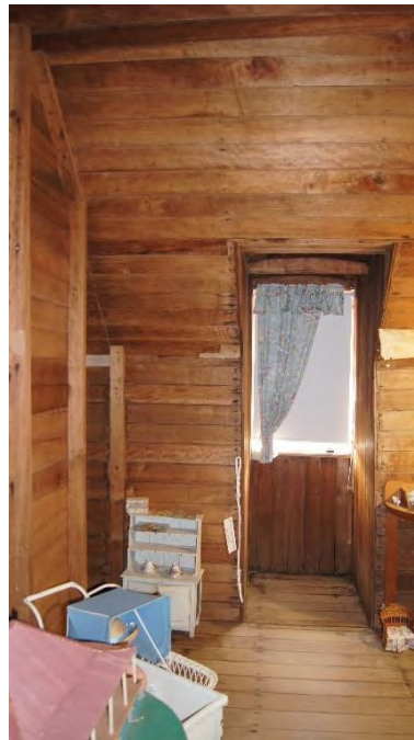
Figure 63: Dormer, double hung sash window along the south western wall of the attic (AHS, 2019).
