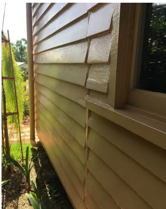
Figure 30: South eastern external wall showing the division between the early enclosure of the western verandah and the 1930s verandah enclosure (AHS, 2019).
