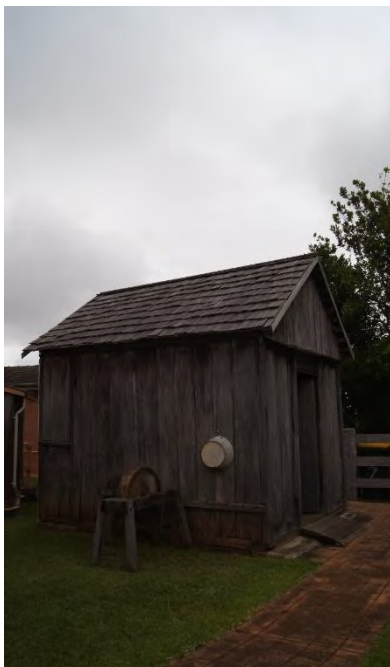
Figure 19: Slab hut with shingled roof (AHS, 2019).
