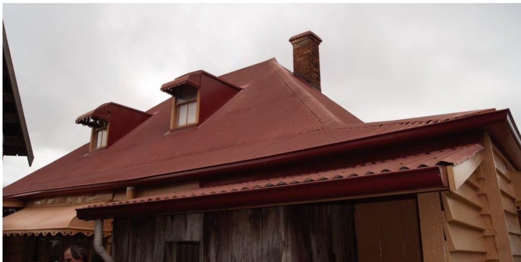
Figure 23: South western side of the roof showing chimney and barrel roofed dormer windows with hoods (AHS, 2019).
