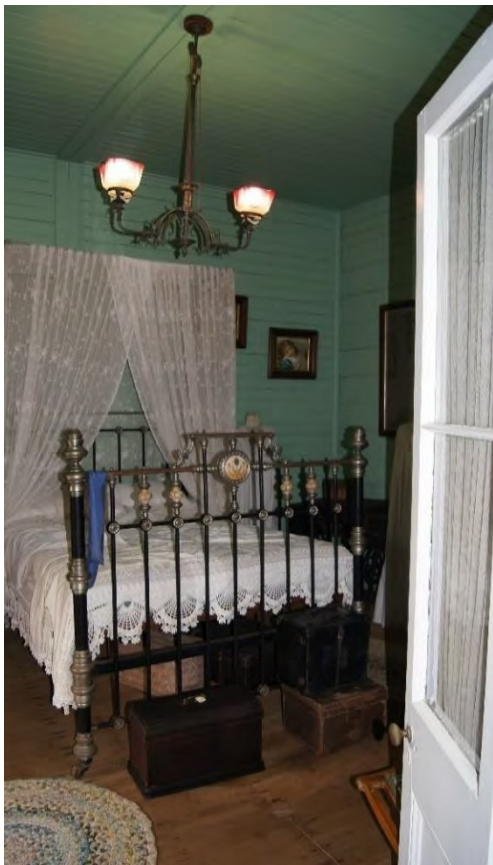
Figure 47: Bedroom looking towards the north eastern wall showing later addition wall and ceiling VJ board lining (AHS, 2019).
