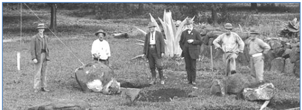
Building a new bowling green near Captain Burrows' house in 1919 (See below). Note the large boulders that had to be removed to get a level surface. Almost certainly Captain Burrows on the left. Photo taken from Burrows' house. Thanks to Mark McCudden for this image which originally came from the Queensland State Heritage Library.
